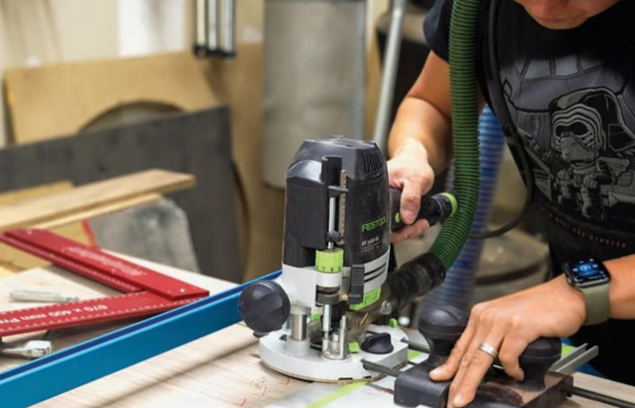
Use a 3/4" straight bit (or a 23/32" undersized plywood bit if your stock isn't a true 3/4") to plow matching 1/4"-deep dados across the top and bottom panels to house the large vertical partition.
