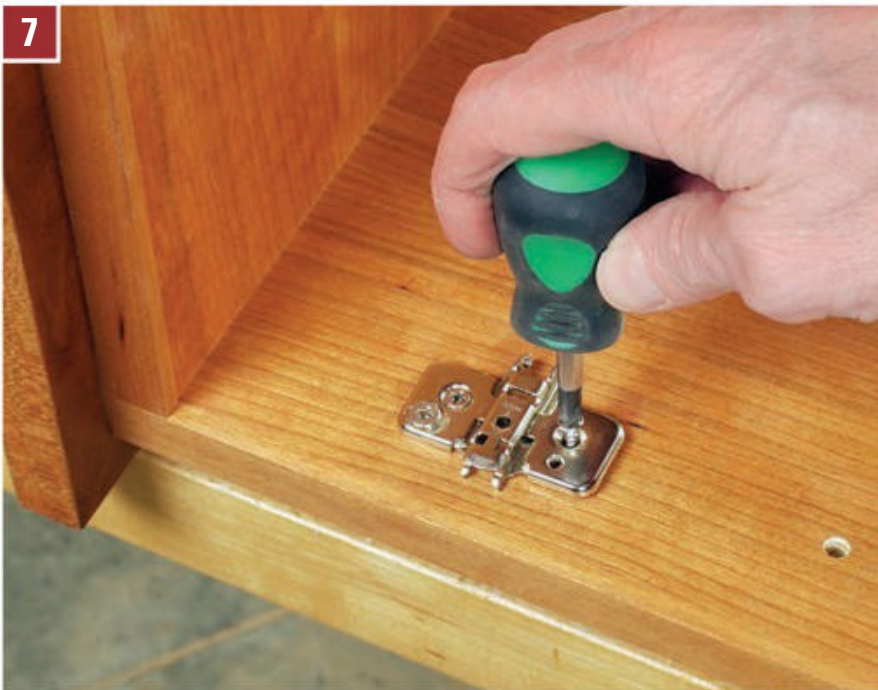
7 With long-arm style Euro hinges like these, the mounting plates are installed independently of the rest of the hinge hardware. Fasten the hinge plates to the cabinet with their attachment screws.
