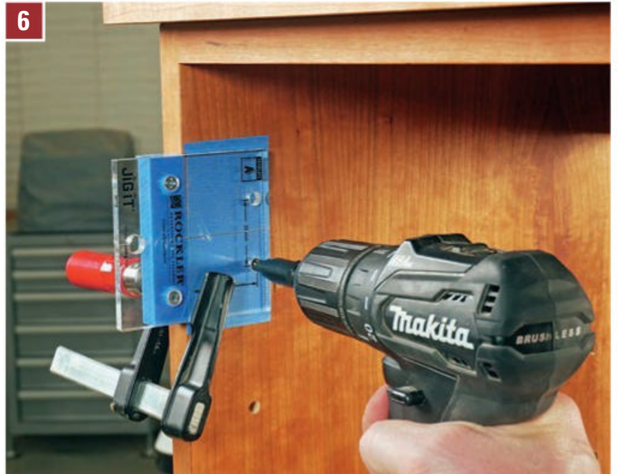
6 Locate and drill pilot holes for pairs of screws that will attach the hinge mounting plates to the cabinet. Here, Rockler's JIG IT Mounting Plate Template "A" sets the screw placement and setback without measuring.
