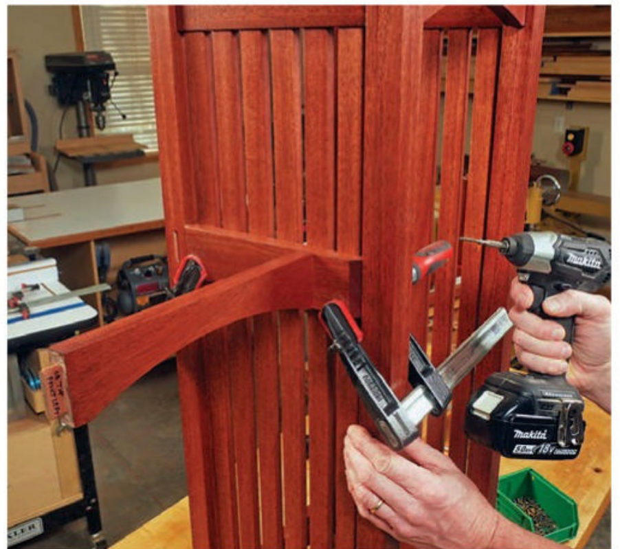
Attach the cross rail to the top front rail of the outer assemblies with 2" countersunk wood screws. Then clamp that assembly in place in order to fasten the cross support and outermost slats together with #6 x 1" screws.
