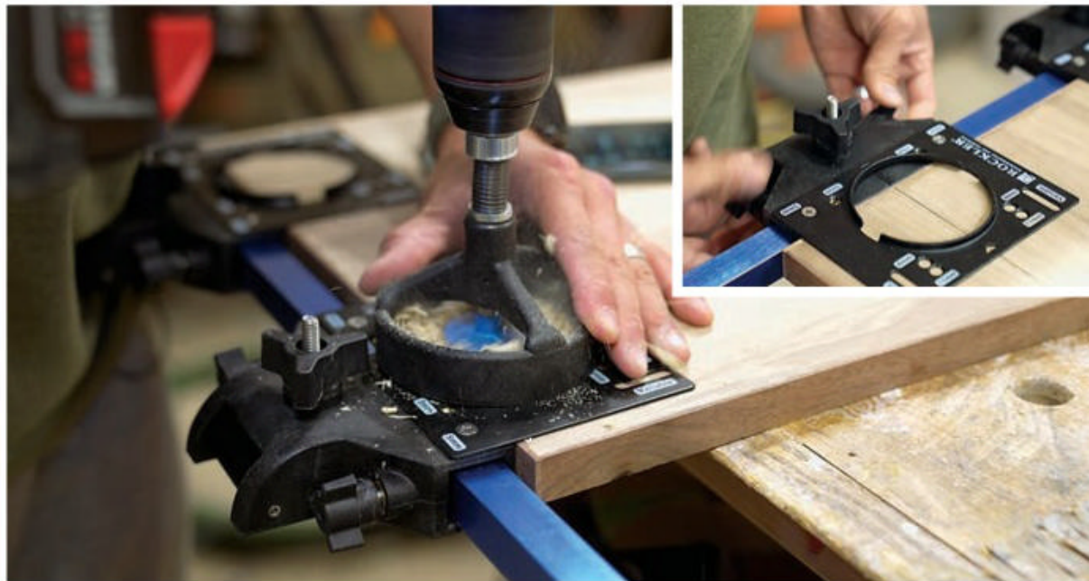
Bore a pair of 35 mm stopped holes in the back of each door for the hinge cup hardware. Here the author is using Rockler's JIG IT Deluxe Concealed Hinge Drilling System, which sets the spacing of these mortises and allows them to be bored with a handheld drill.
