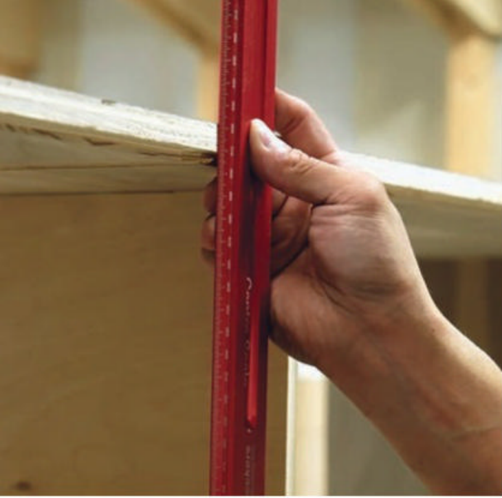
While the Material List provides the length of the large vertical partition, it's always a good idea to measure off of your actual project (left) to verify captured part lengths like these. Once it's cut to size, notch the front corners of the partition so it fits into and around the carcass dadoes (center, right photos). All three of the carcass's partitions and horizontal shelf will be notched this way.
